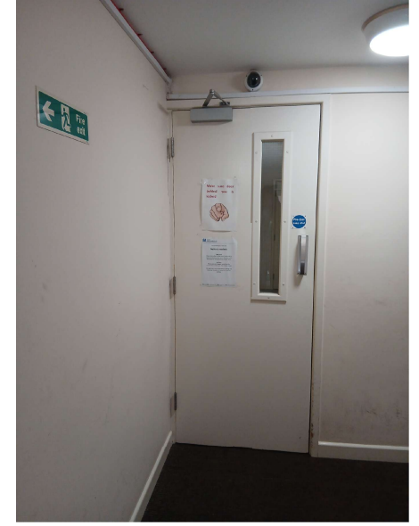
Internal Doors (Compartment Doors)
